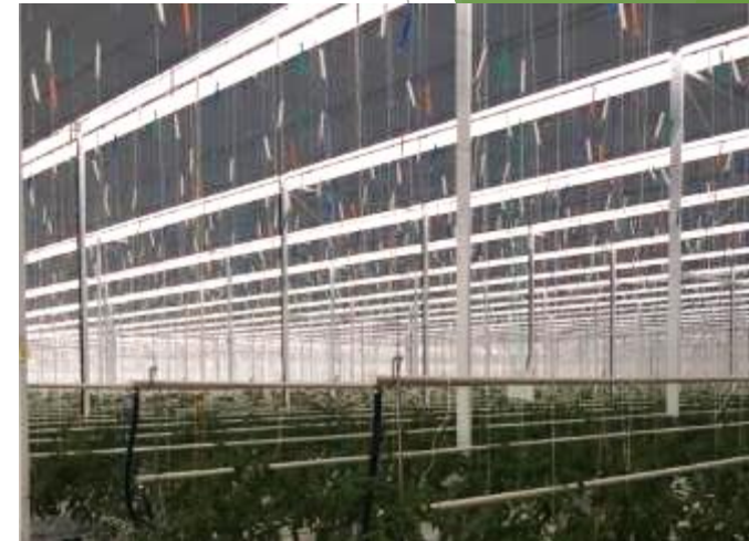
Thermal screens on roof
