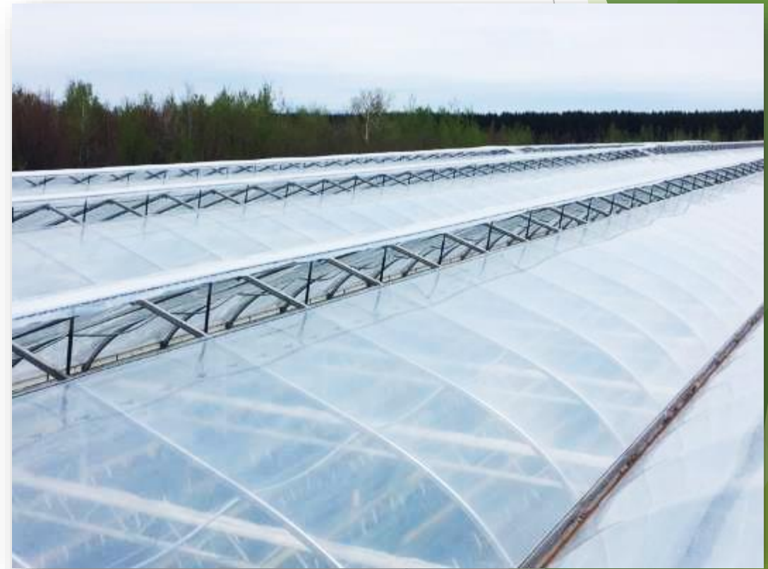
Double polyethylene open roofing
