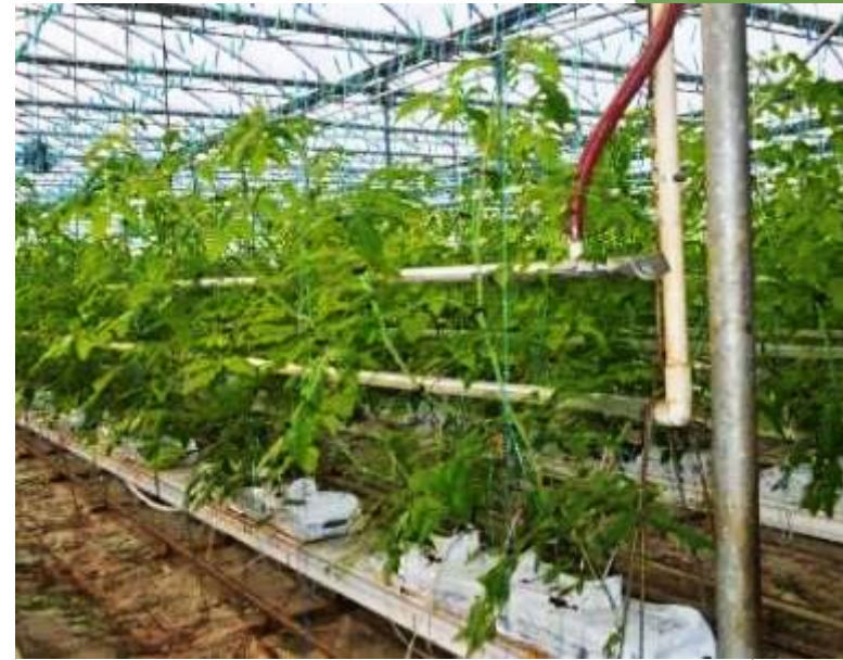
CO 2 distribution via hose
