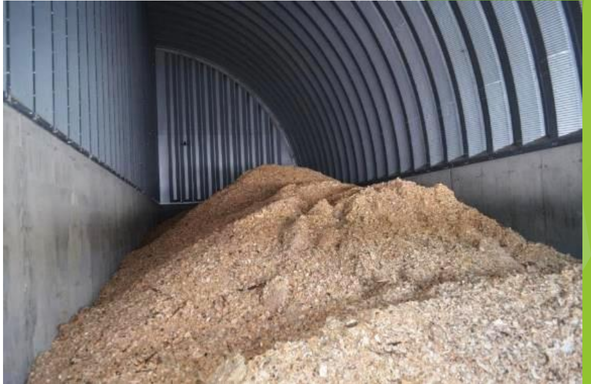
Wood chip storage
