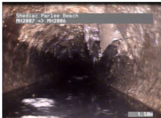
Figure 2-4 Sewer video sample of section near Lift Station.
