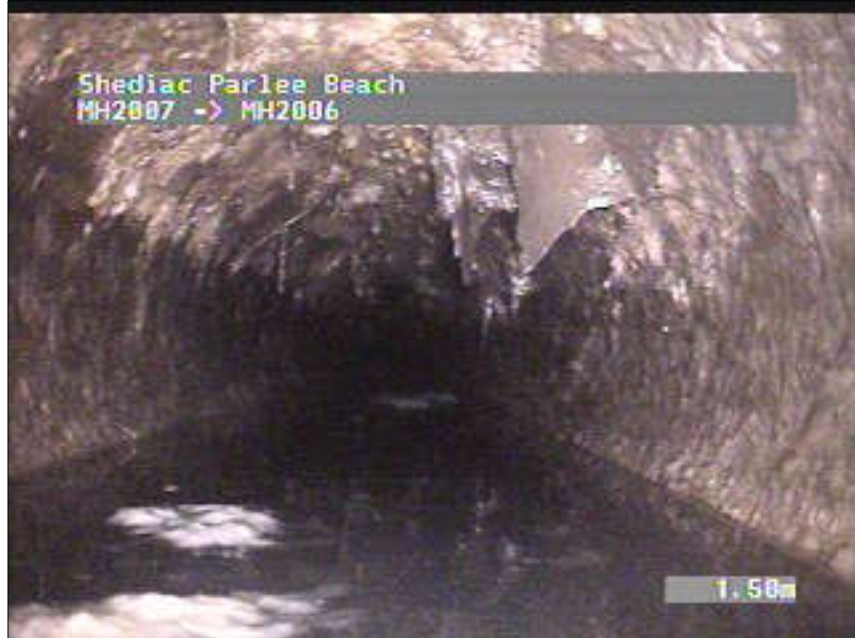
Photo: 7_7_63_A.JPG, VCR No.: 2 1.5m, Survey Abandoned
