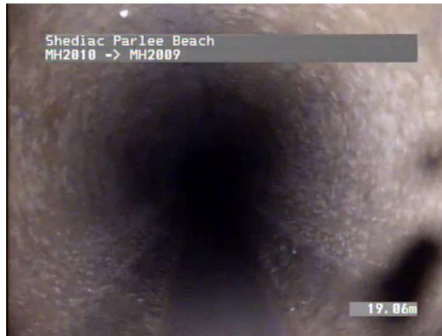
Figure 2-3 Sewer video sample of section in the dunes.
