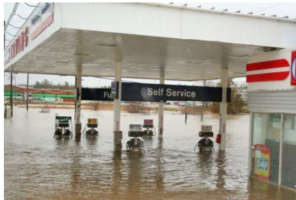
Figure 2 An Irving gas station was filled with flood waters in December 2010. Source: Jennifer Pritchett, Telegraph-Journal, December 15, 2011
