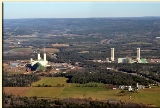
Figure 4. Photograph of PotashCorp's existing Penobscis facility (left) and construction at their new Picadilly facility (right) in southern New Brunswick near Sussex.
