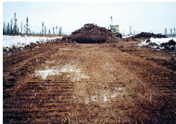
Figure 8. Stacking plant material collected on frozen ground.
