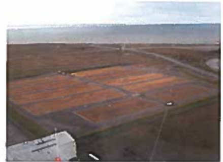
Aerial view of system
