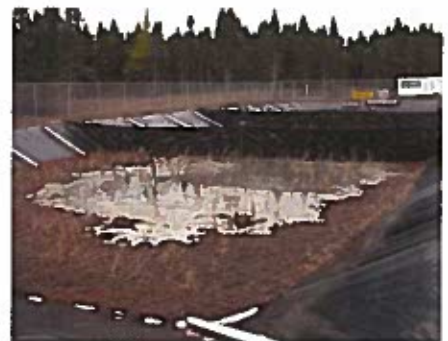
Sludge treatment cells
