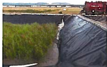
Application of sludge to sludge cell
