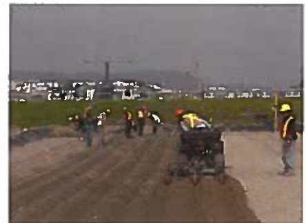
Planting during construction
