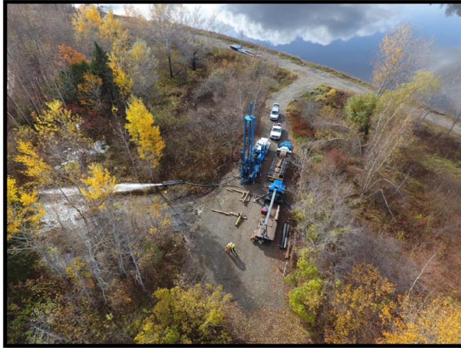
Photo 1: Looking down onto the production well area during water exploration activities.
