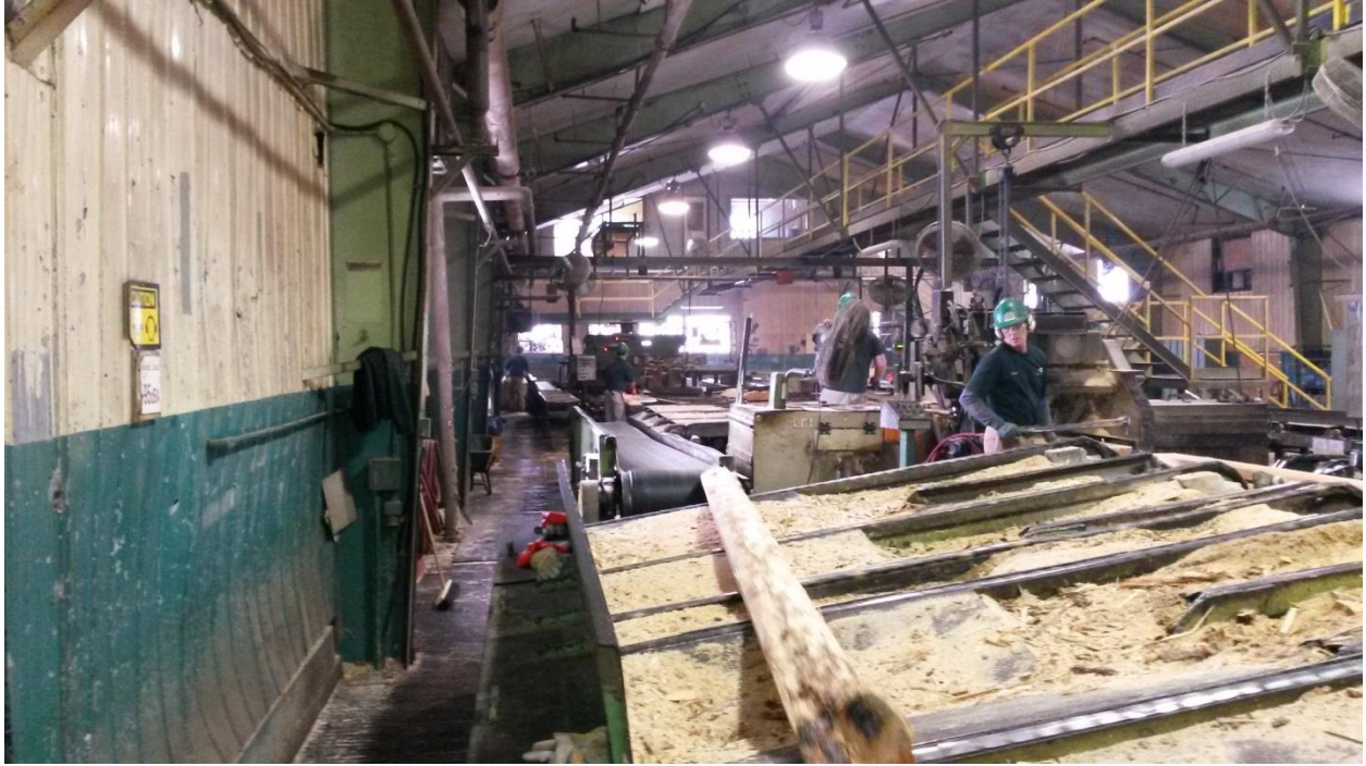
Photo 15. Sawmill interior, upper level.
