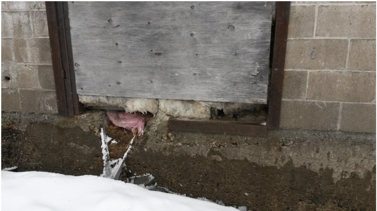
Photo 10. Exterior brick wall and concrete foundation of sawmill building.
