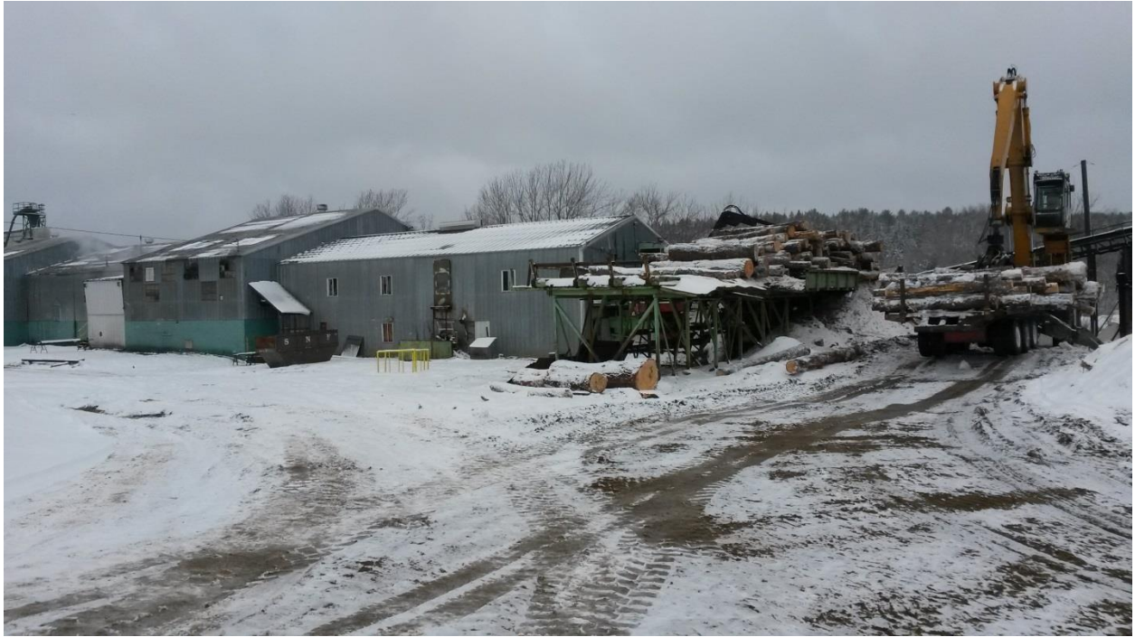
Photo 5. Sawmill structure looking north from yard.
