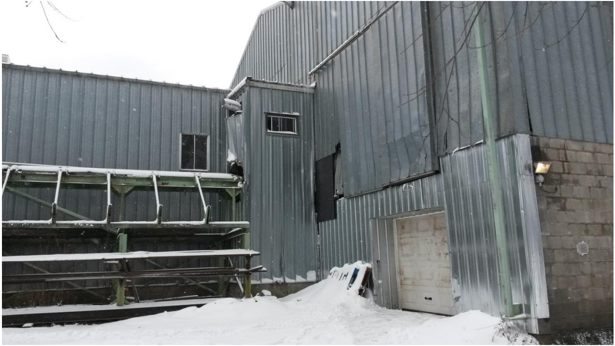
Photo 9. Exterior metal cladding on sawmill building.
