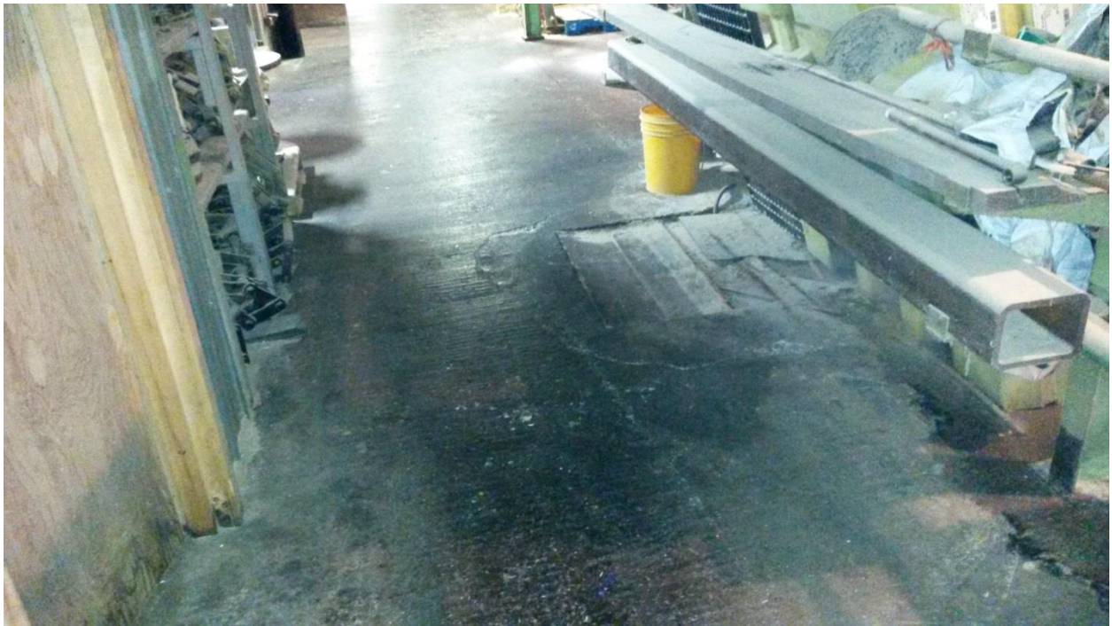
Photo 12. Sawmill interior – concrete floor, sawmill lower level.
