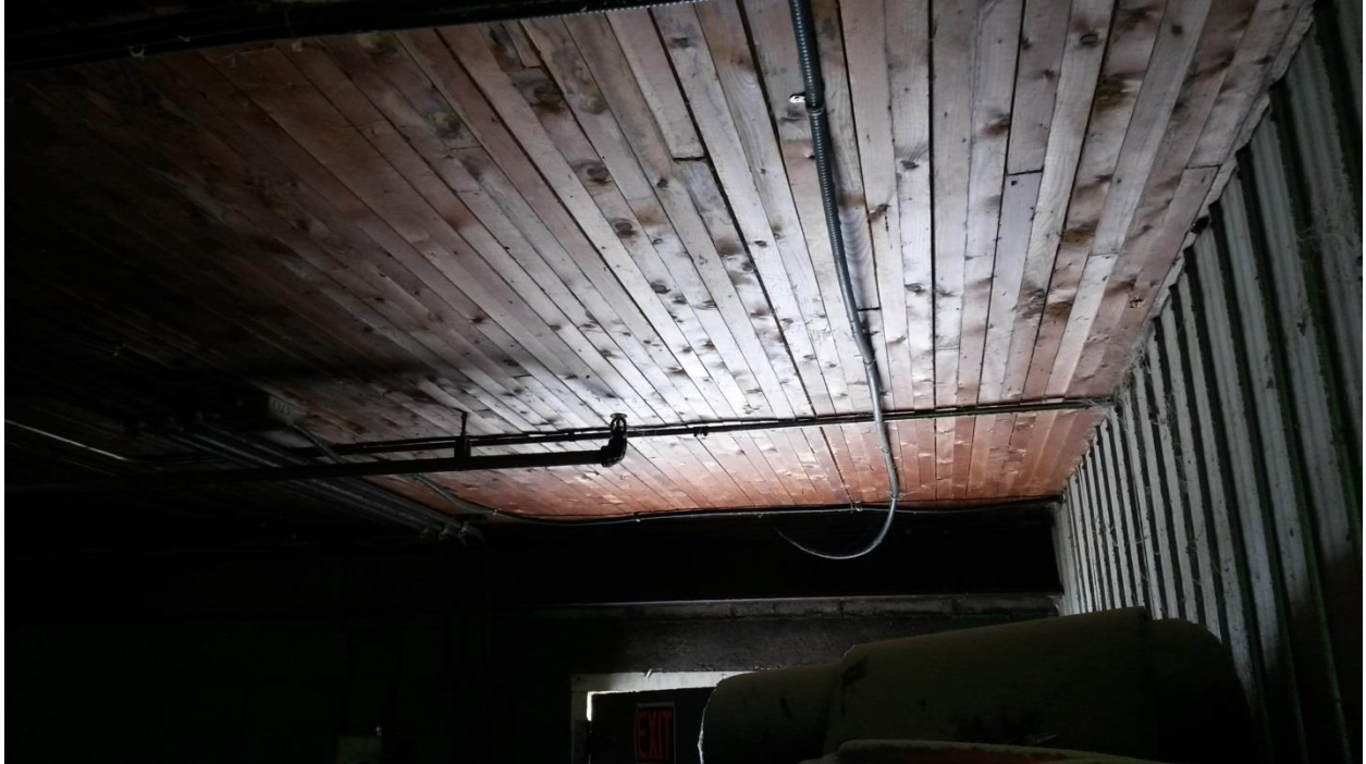
Photo 11. Sawmill interior – roof of lower level/upper level floor (wood).
