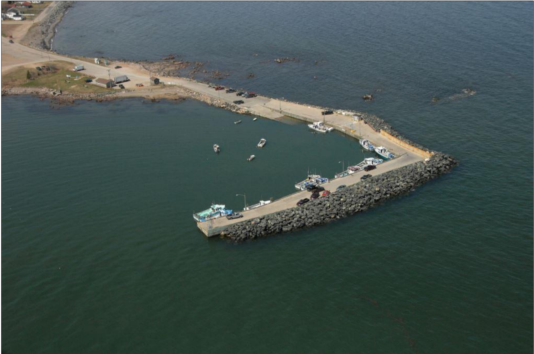
Figure 3: Oblique aerial photo of Petit-Rocher DFO-SCH, Gloucester County, New Brunswick
