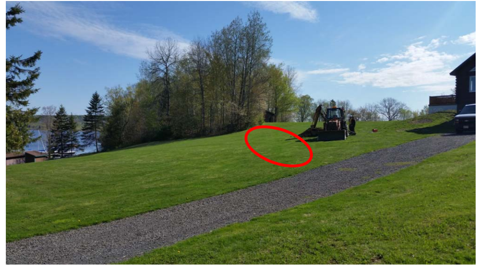
First contour trench location
