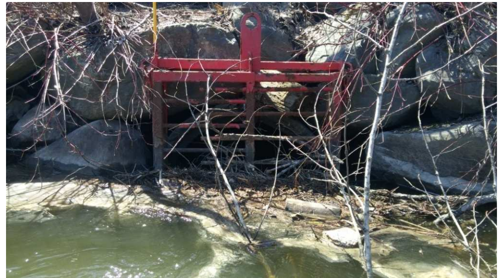
Upstream end of culvert
