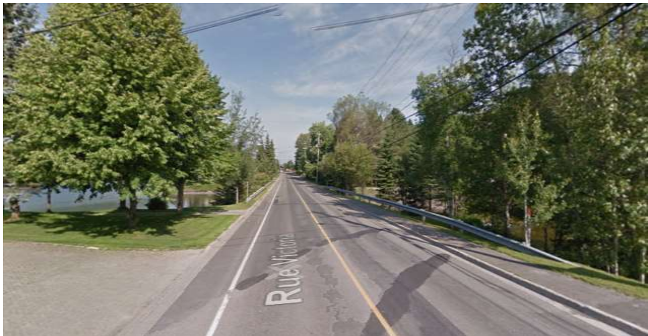
Photo No. 1: Victoria Street at McRae Brook (Google Earth)
