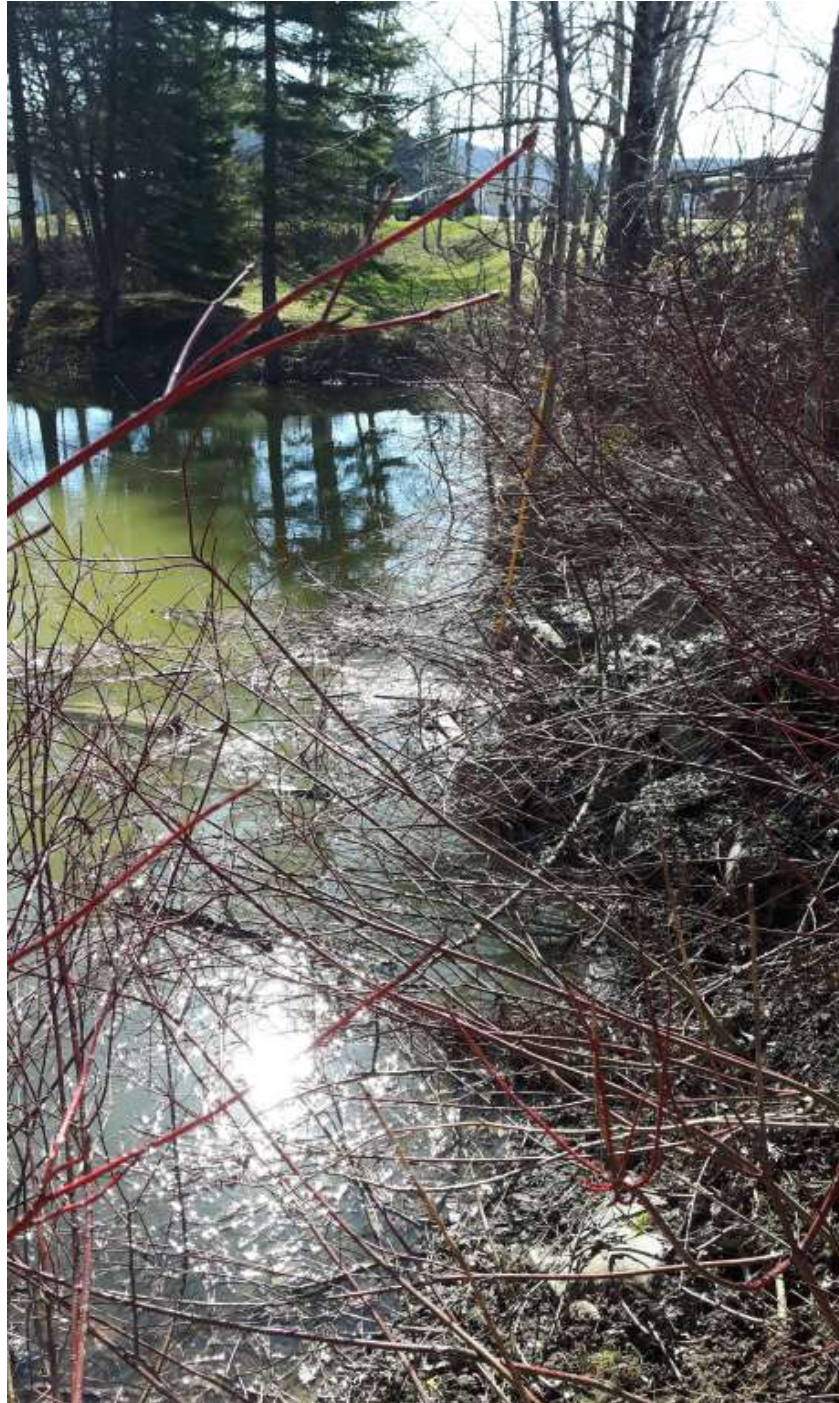
Photo No. 2: Upstream Side of Victoria Street Culvert
