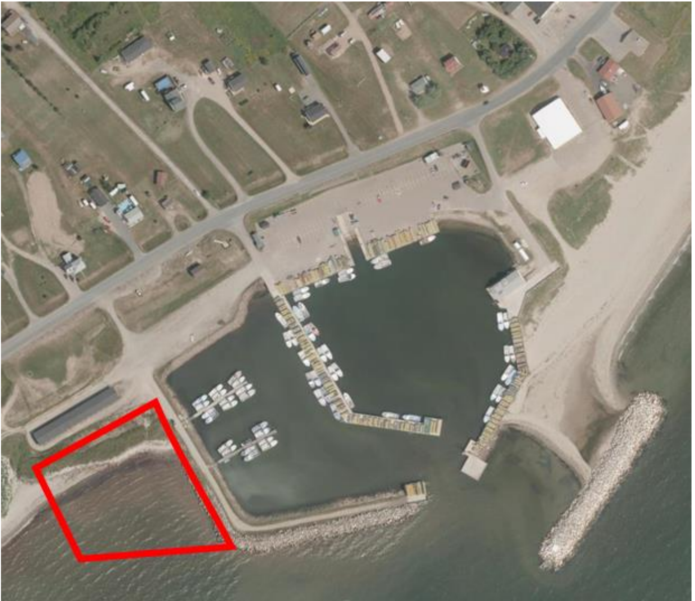
Figure 3: Aerial view of Pointe-Sapin SCH with location of proposed containment cell indicated in red.
