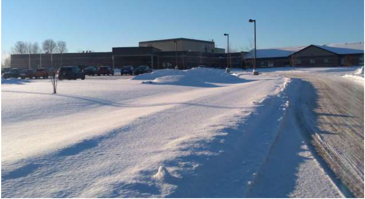
Photo 1: General View of Nursing Home Building Looking South (November 22, 2018)
