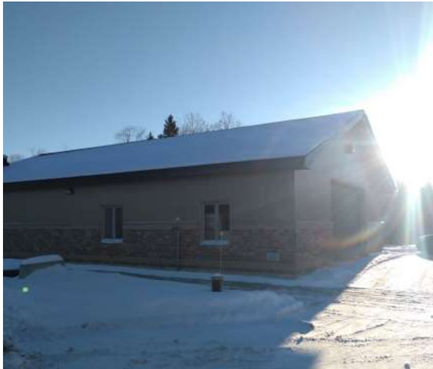
Photo 2: View of Well No. 1 (November 22, 2018)
