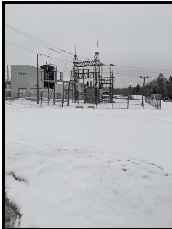
Photo 4 – Existing infrastructure and proposed excavation area facing east
