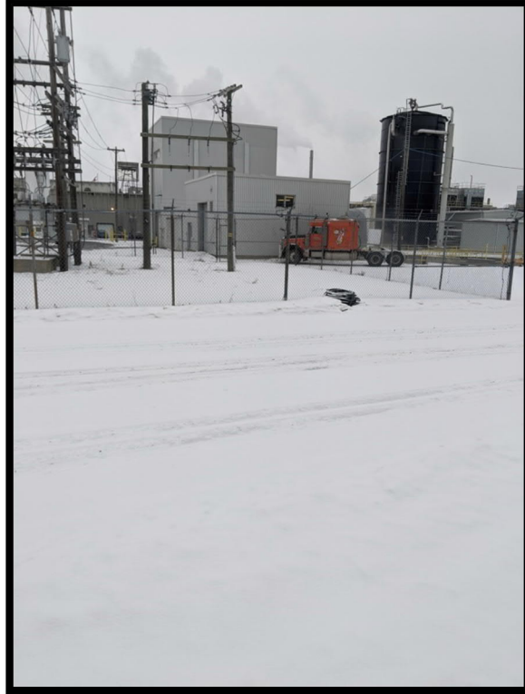
Photo 3 – Existing infrastructure and proposed excavation area facing northeast.
