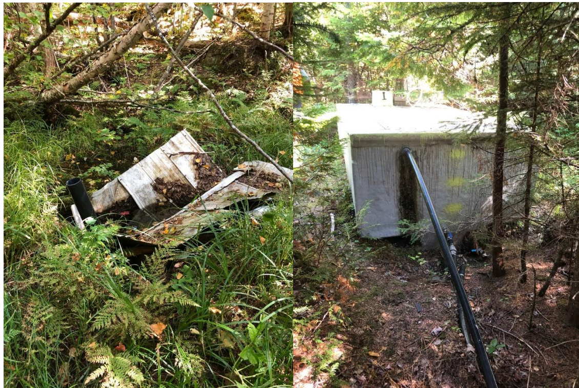
(a) Spring water intake
