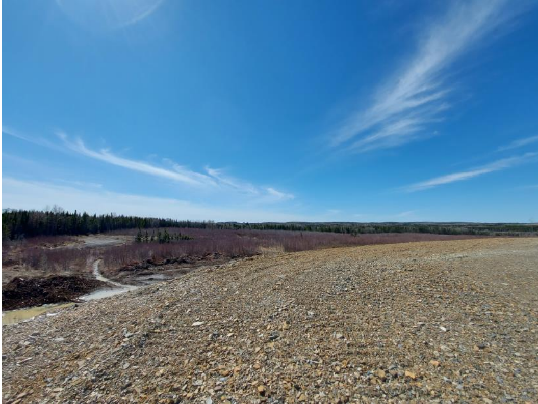
Photo 5. Taken from southwestern edge of capped C & D cell, facing west.
