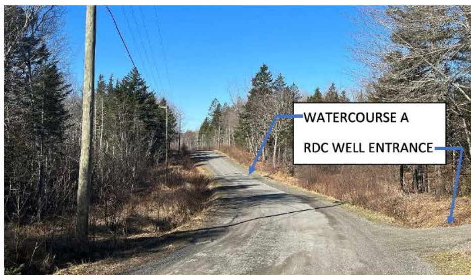
Figure 4 - Chamcook No. 3 Rd at RDC Well Entrance
