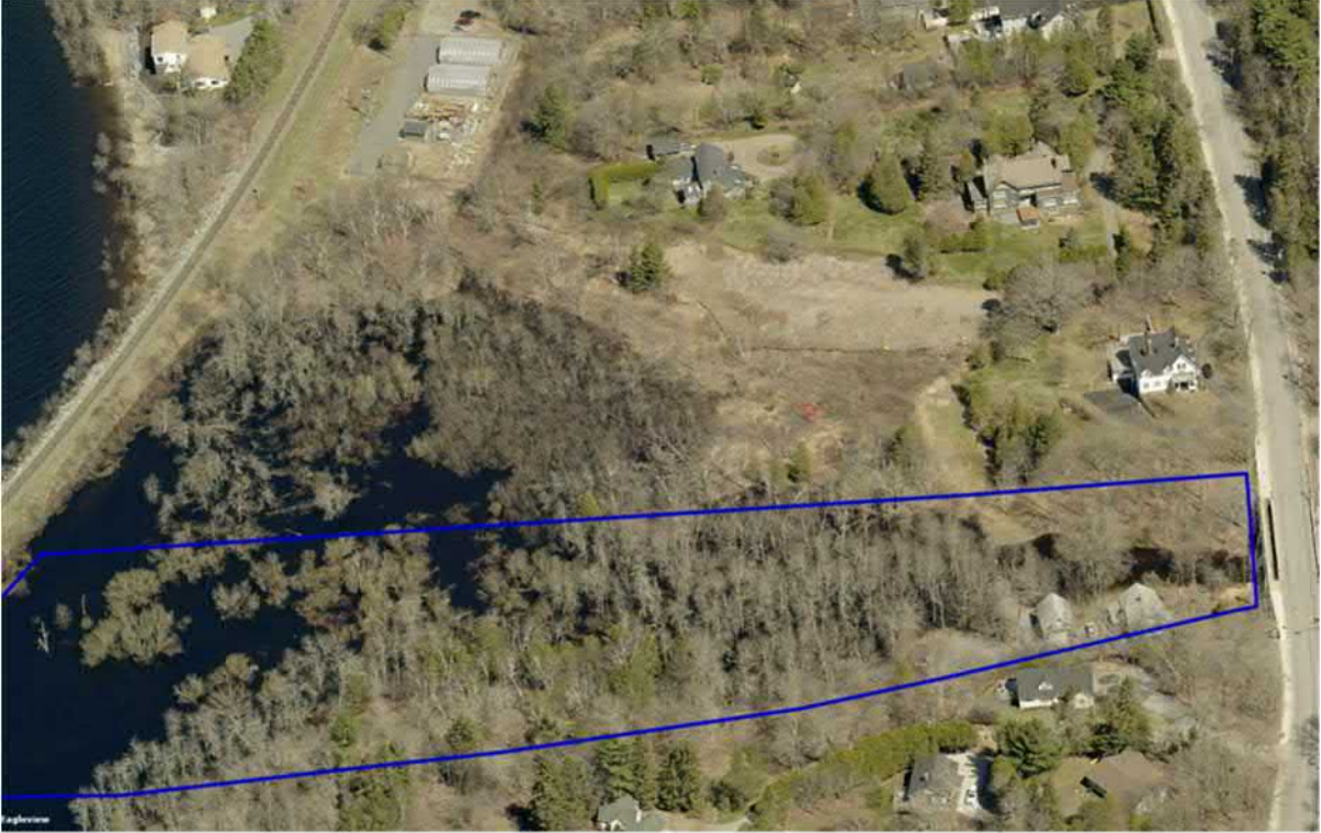
Photo 1. Aerial imagery depicting spring flood conditions at the study area (NBDELG 2020). Date of imagery unknown
