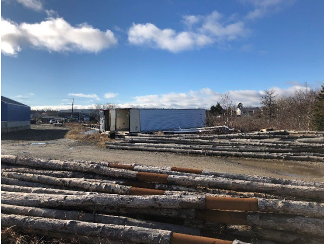
Photo 1: View of Section A looking in the west direction.
