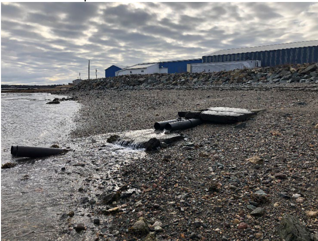
Photo 25: Four pipes from fish plant in Section C. Note two pipes are discharging while other two were inactive at the time of the Site visit.
