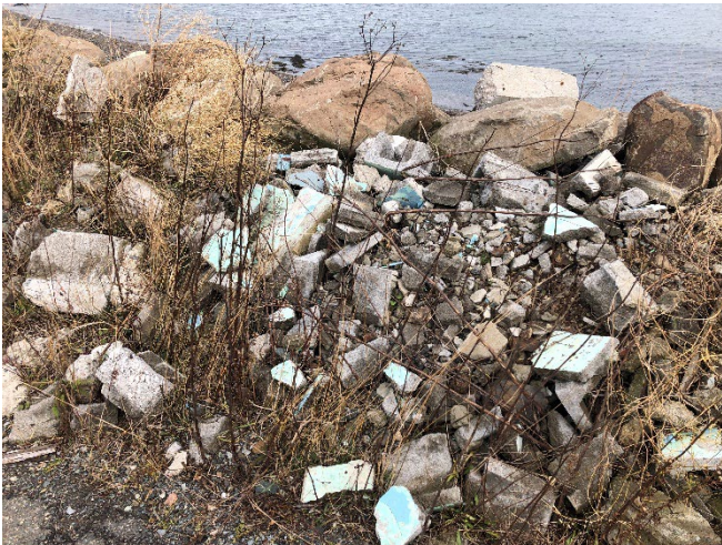
Photo 21: Cement debris present within the berm along Section B.
