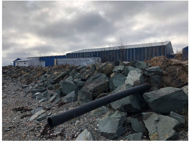
Photo 20: Potential stormwater drain pipe along Section B.
