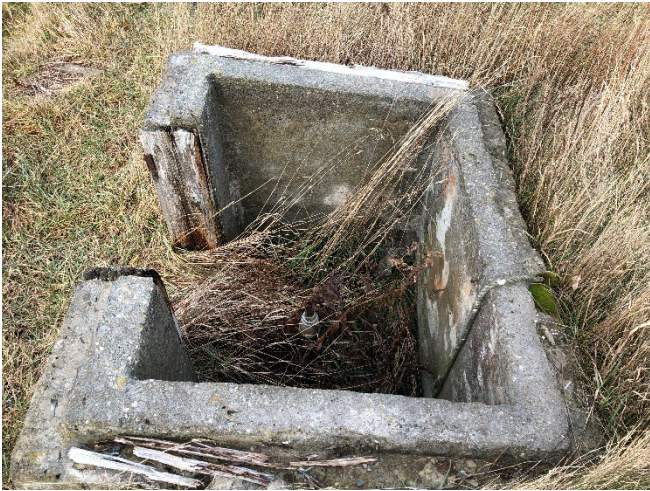
Photo 19: Well near Section B.
