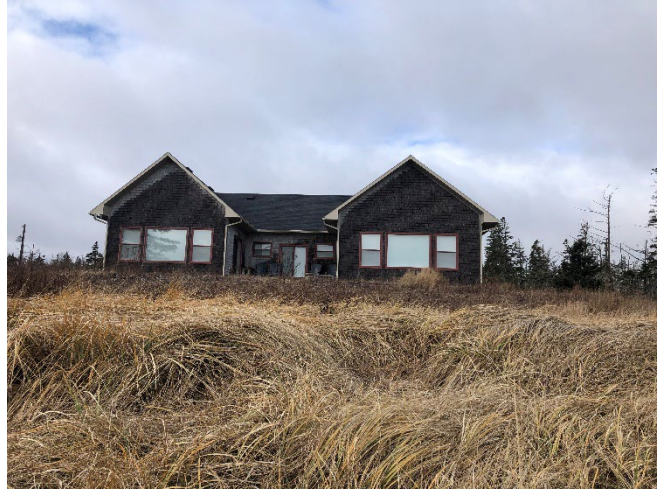
Photo 8: Residential building (PID No. 15164775) near the north end of Section B looking to the west.
