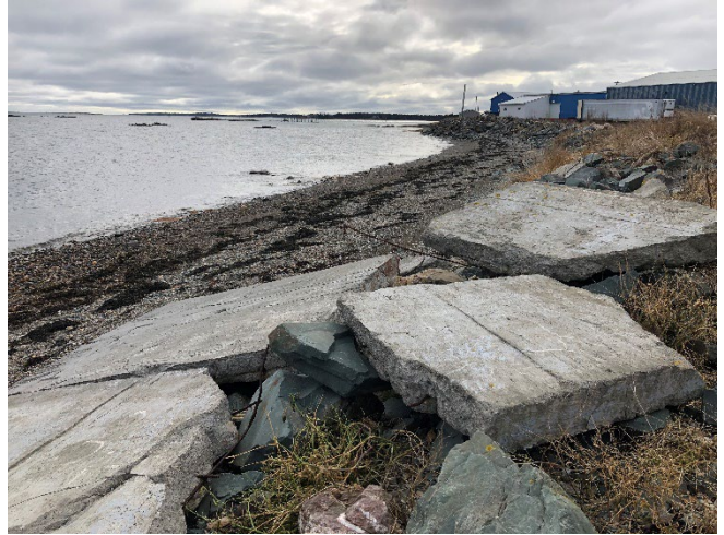
Photo 18: Cement blocks on Section B looking south.
