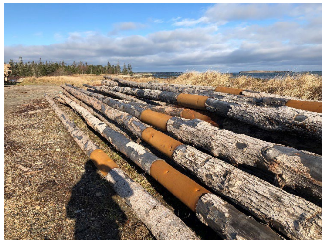
Photo 6: Wood poles stored in the laydown area of Section A.
