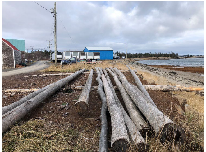
Photo 22: Fill material under wood poles near southern portion of Section B.
