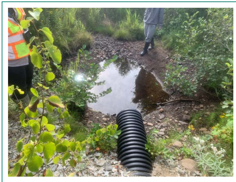
Photo 10: View of culvert on PID No. 15010267 (August 11, 2022).
