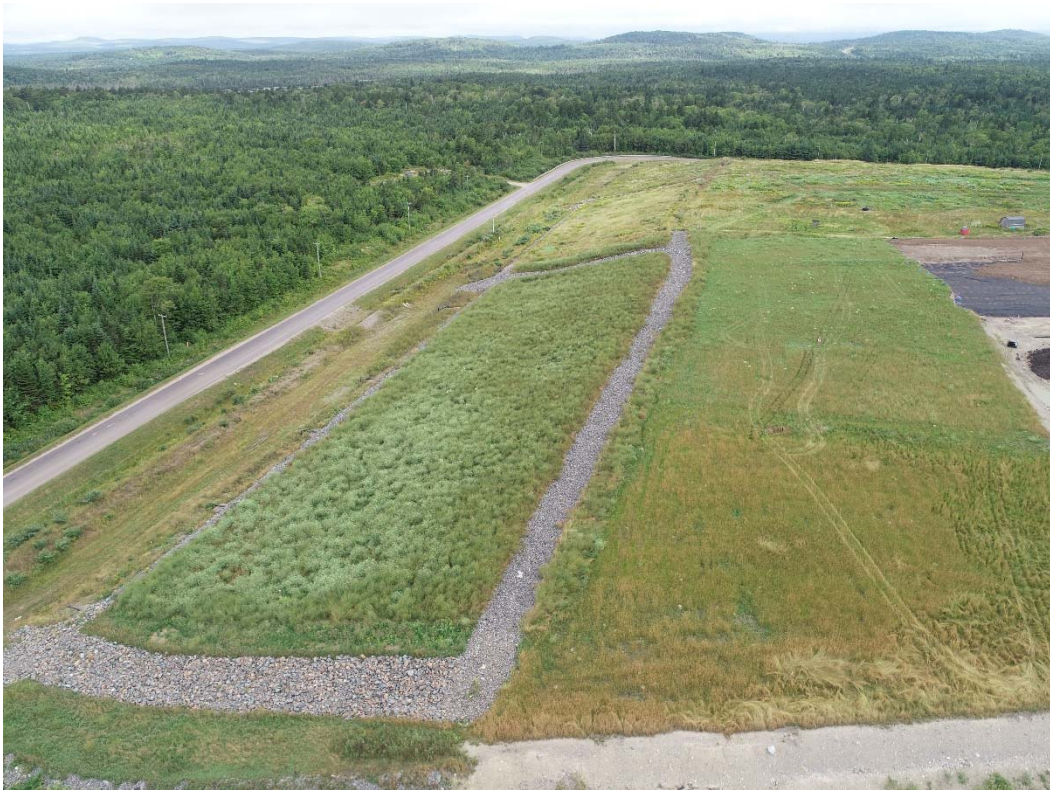
Photo 2: View of final capped landfill containment cells (2023).
