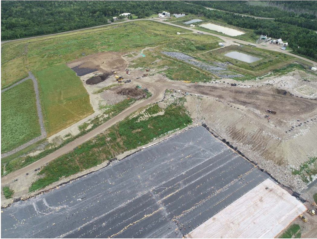
Photo 1: View of capped and active landfill containment cells (2023).
