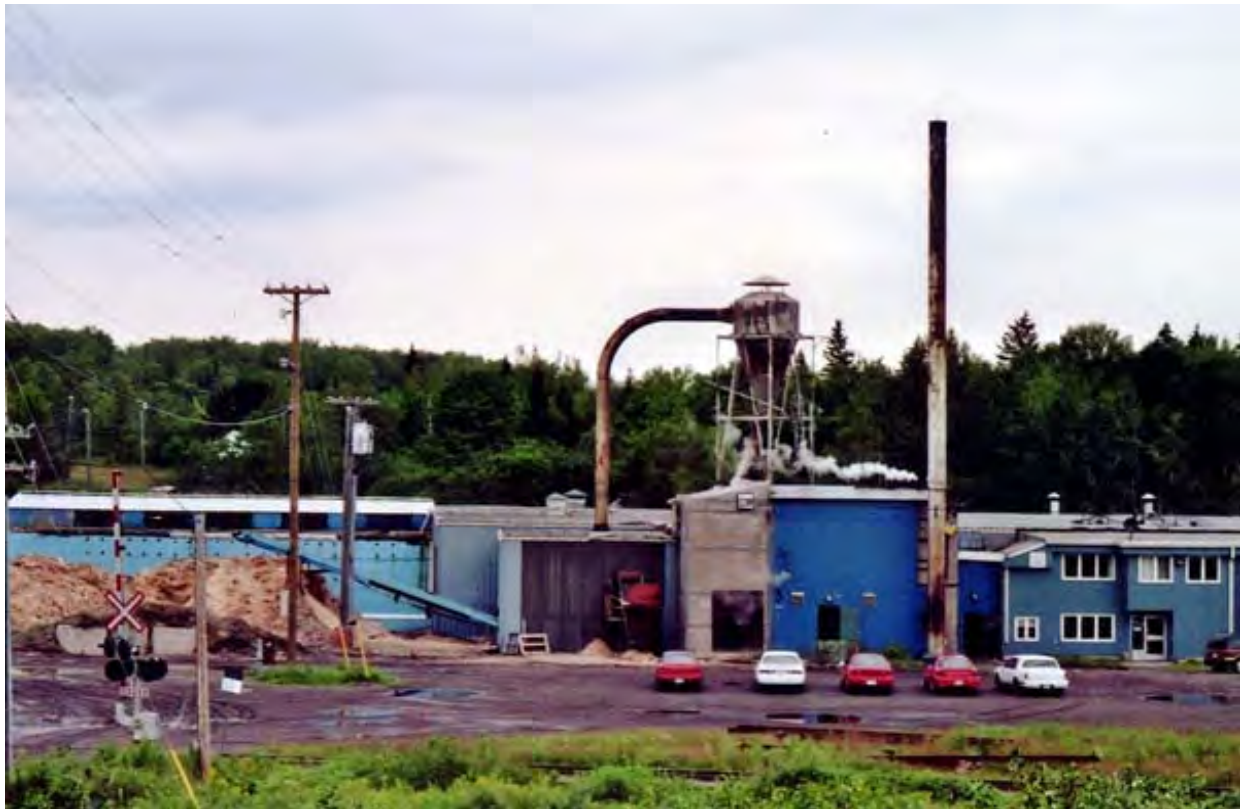
Photo 6.2.9 Atcon veneer mill, Napadogan, New Brunswick (Janice Cook, July 25, 2006). Located on Route 107 between Williamsburg and Juniper, the mill produced veneers for furniture, flooring, doors, skateboards, and musical instrument cases. P194-598 Miscellaneous photographs collection, Provincial Archives of New Brunswick (PANB n.d.).
