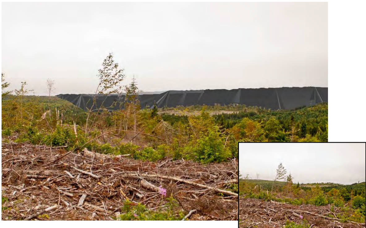
Figure 8.12.11 Modelled View from Within PDA, Looking Northwest Toward TSF (from Photo 2 in Figure 8.12.3, inset)
