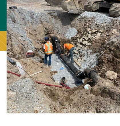
The older pipes were mainly cast iron and replaced most often with ductile iron pipe, a product produced with advanced metallurgy, combining the physical strength of steel and the lifespan of cast iron. Trent Brewer says the first ductile iron pipes went into the ground in Fredericton in 1972 and none have failed to date. He expects these new pipes to last as long as a century before they need replacement.
