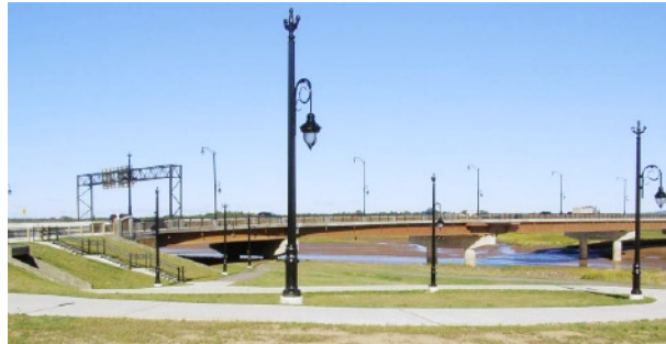
Gunningsville Bridge – Moncton, NB
